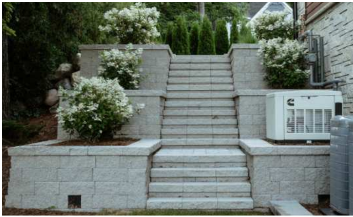
PROJECT INSTALLED BY: DOWN TO EARTH
