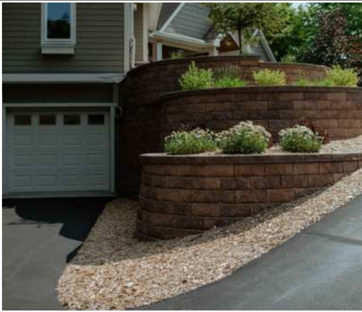
PROJECT INSTALLED BY: DOWN TO EARTH
